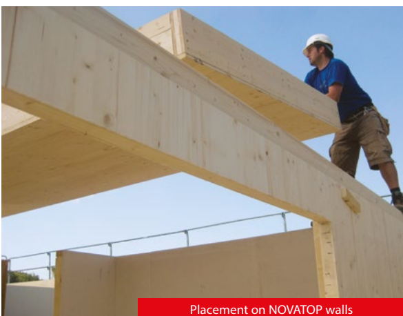
Placement on NOVATOP walls
