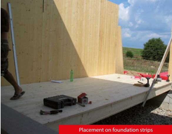
Placement on foundation strips
