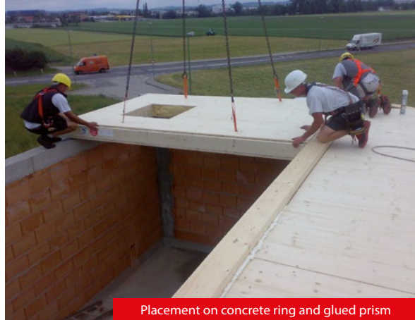
Placement on concrete ring and glued prism
