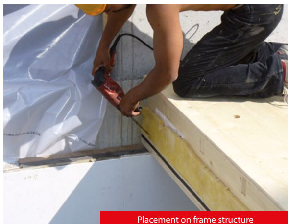
Placement on frame structure
