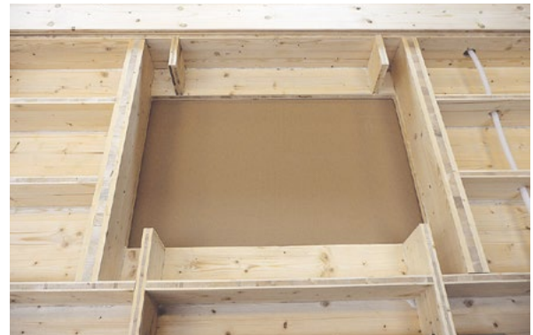
Reinforcement with solid wood at the point of pressure.
