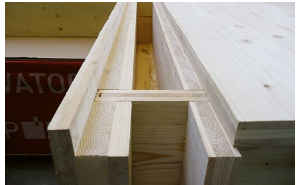
Enclosure of the visual cut-out with a solid-wood panel.
