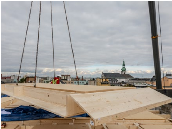
Individual NOVATOP OPEN prefabrication.
