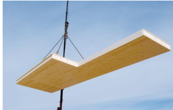
Cut-out in the area of the element over 3 m 2 .
