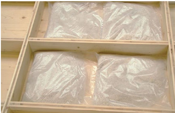
Limestone filling (40, 60, 80 kg/m 2 ).
