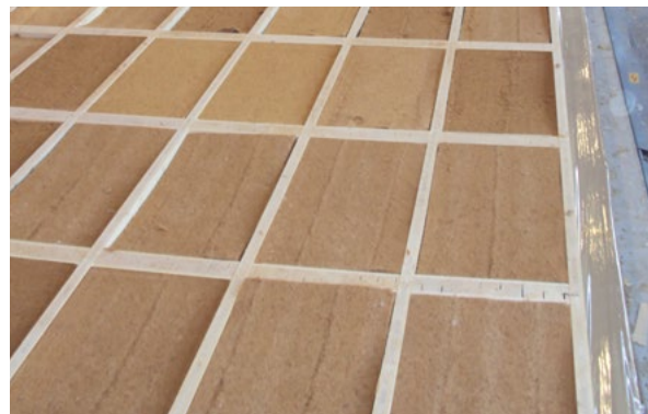
Filling with wood-fibre insulation.
