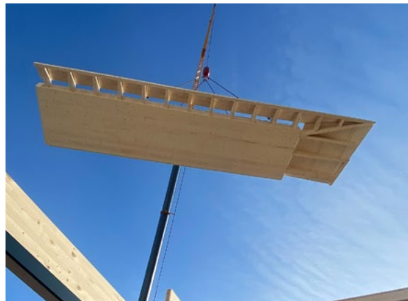
Individual NOVATOP OPEN prefabrication.
