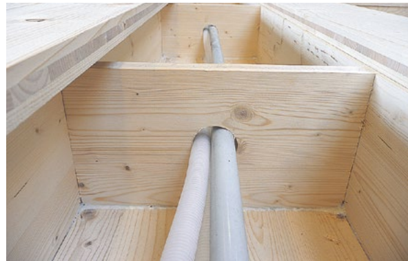
Drilling of holes into the ribs for wiring and piping installations.
