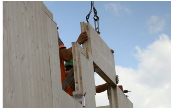
Preparation of connection and installation – SOLID 84, 124 mm.
