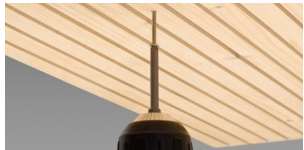
Screws in the area of the panel
